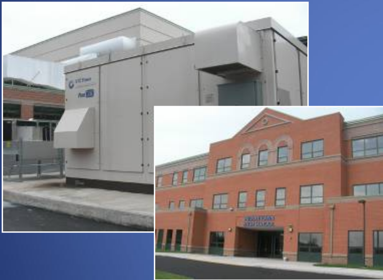
200 kW UTC Power Fuel Cell
